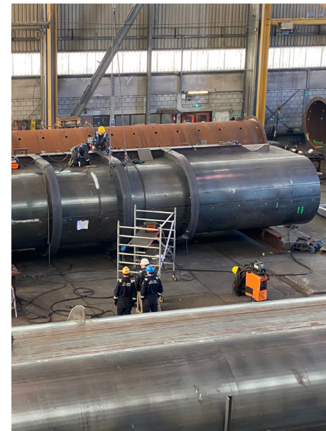
Figure 30: Production of a switch guideway segment.
