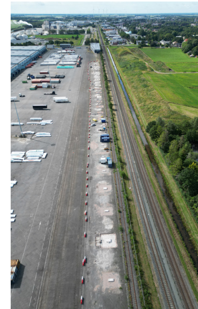
Figure 31: On-site aerial photo of the EHC during substructure construction.
